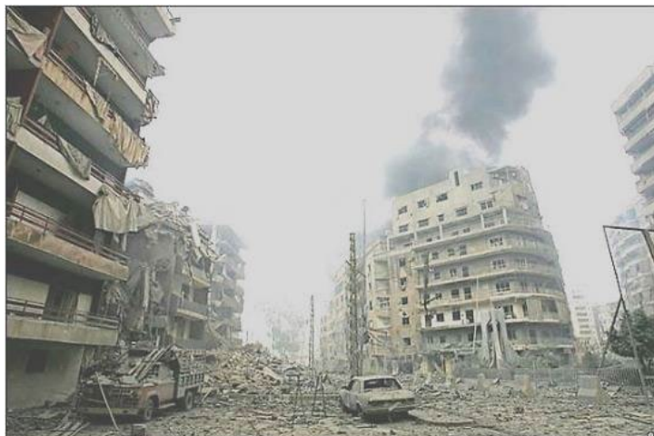
Figure 20: Example of MDZ-Like Blast Damage
